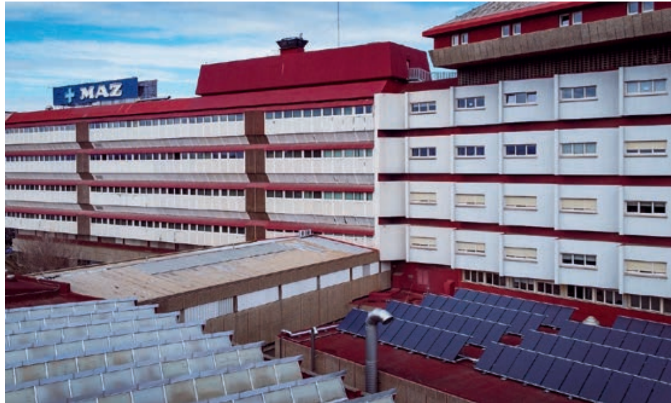
Zaragoza - Installation of hybrid solar panels in La Maz hospital
