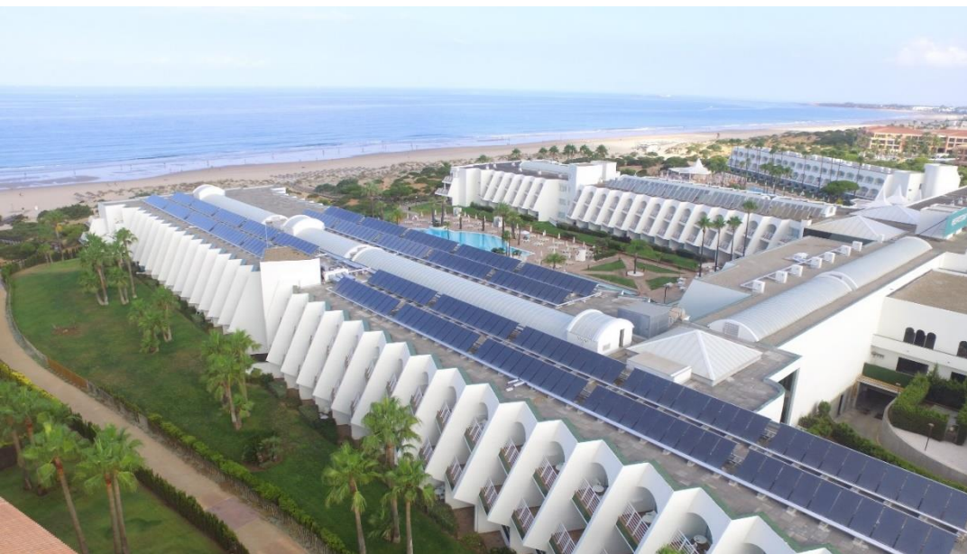
Installation on the roofs of the Iberostar Royal Ándalus Hotel, Chiclana (Spain)
