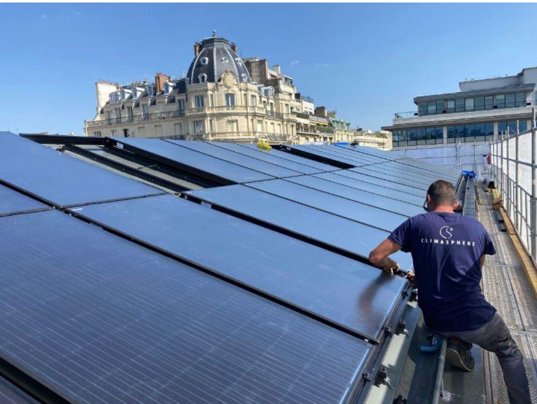
Installation at the OECD, Paris (France)
